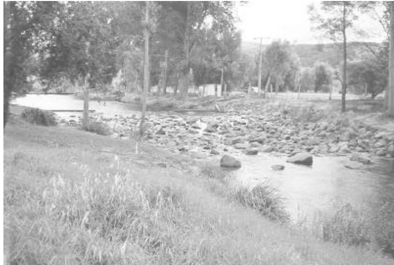
Figure 1: Prototype Fishway Installation.
